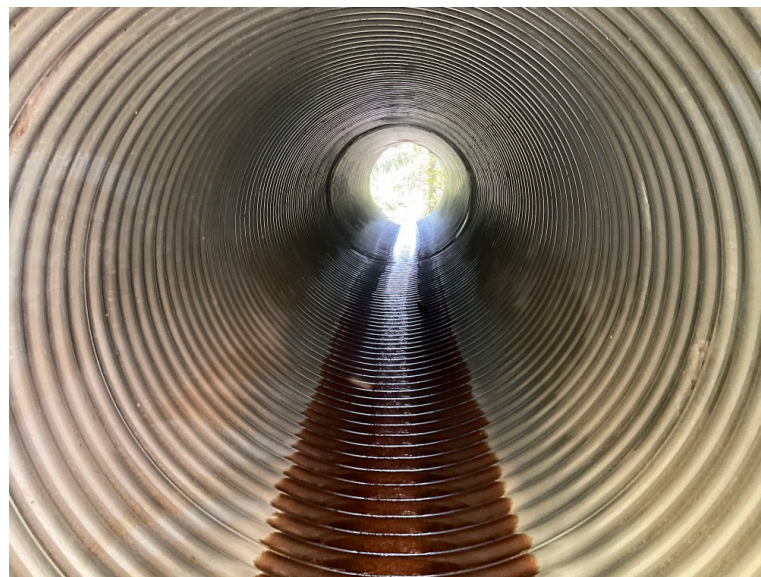
Looking Downstream Through CMP
